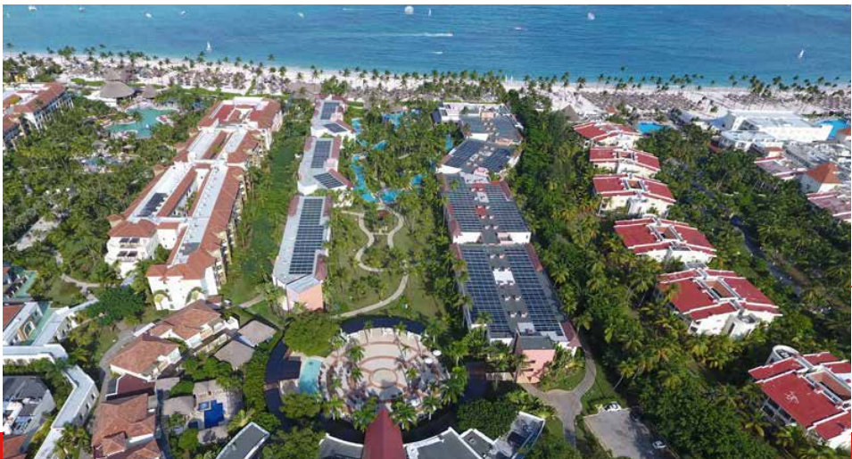
1.2 MW Dominican Republic
